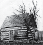
Gardner cabin, Douglas County
